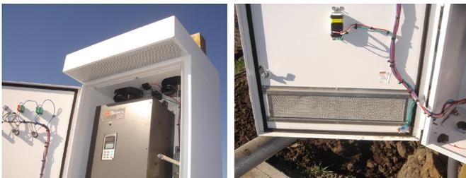
*White panels and ventilation are used to reduce heat loads for VFDs. Air is drawn from the bottom of the cabinet (right) and exhausted through the top. Fans are thermostatically controlled, but the filters need to be periodically cleaned for everything to work properly.*
