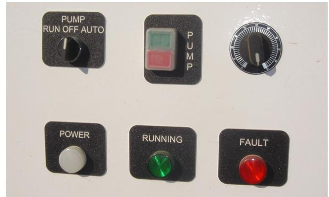
*VFD pump panel controls. Auto (sensor driven) or manual mode (upper left), start/stop (top center), variable speed dial (upper right), power to panel indication (lower left), VFD operational indication (bottom middle) and fault indication (lower right).*
