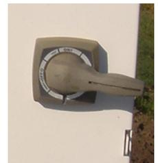
*Safety shutoff/lockout for VFD panel.*
